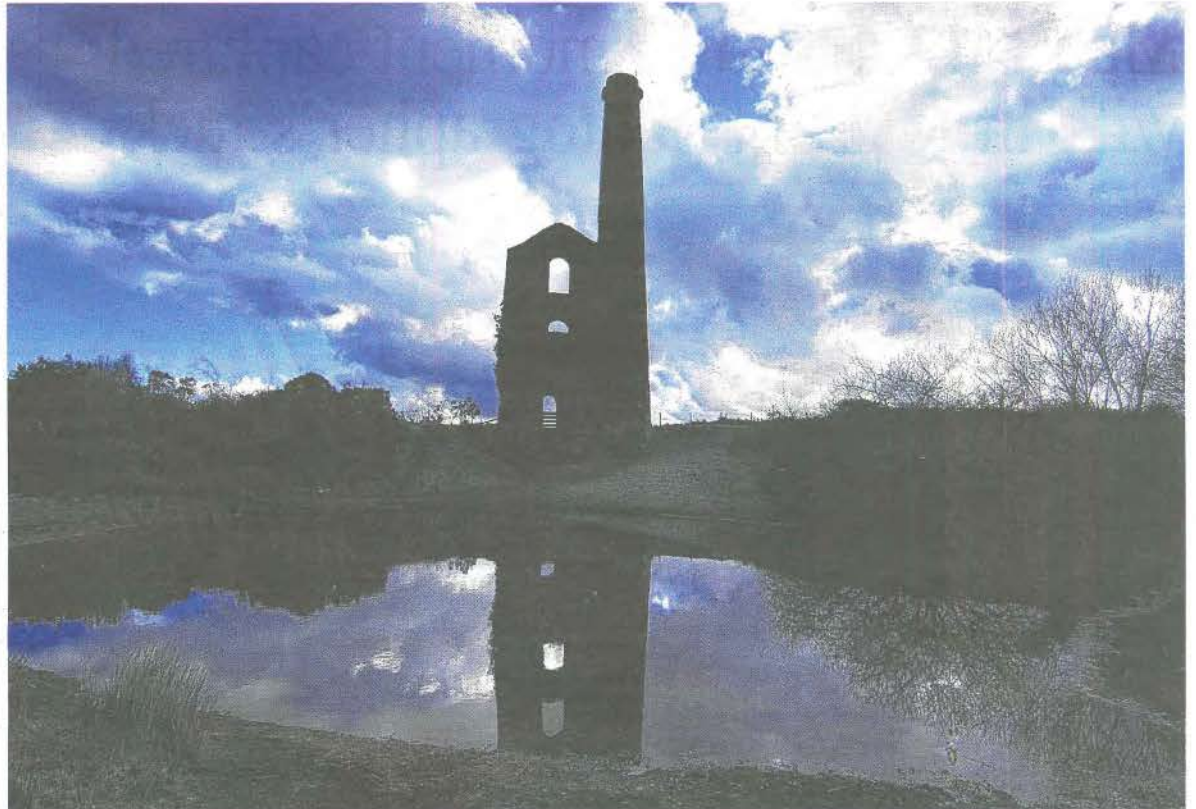
The remains of an old mine engine house in the United Downs area of Cornwall, symbol of the past prosperity of the region that the South West Charter seeks to rebuild
